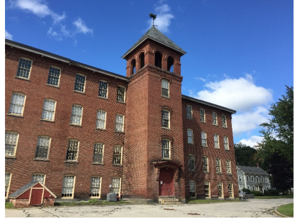
Former Colony Worsted Mill, also known as Abbott Mill Image Credit: Wilton Planning Board & NRPC
