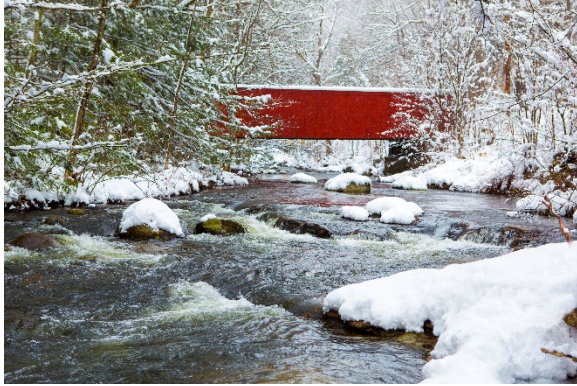
Livermore Bridge over Blood Brook Image credit: Liesl Clark Photography
